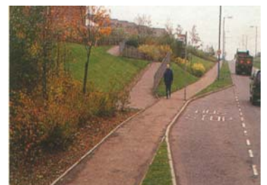
Ramped access to bus stop
