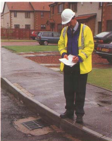
Two stage completion inspection
