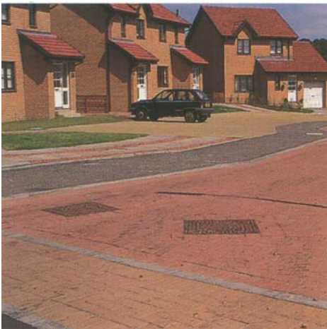
Sewers under Carriageway
