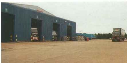
Loading and Parking Manoeuvrability
