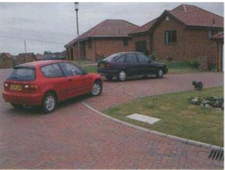
Private Residential Driveway
